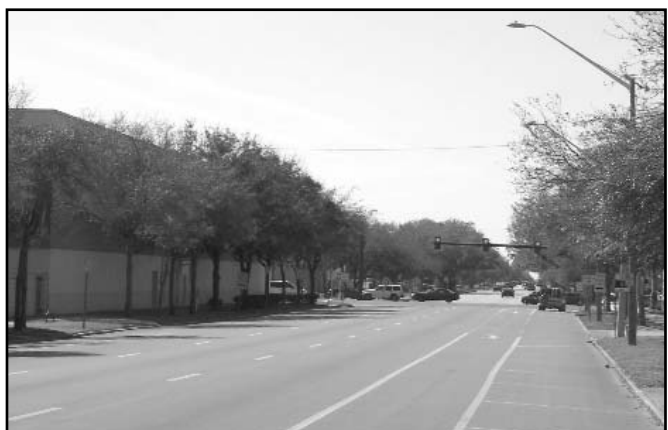
Bicycle Lanes on 1st Avenue N east of 34th Street
