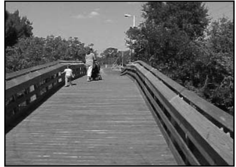
New bridge on Rio Vista Trail
