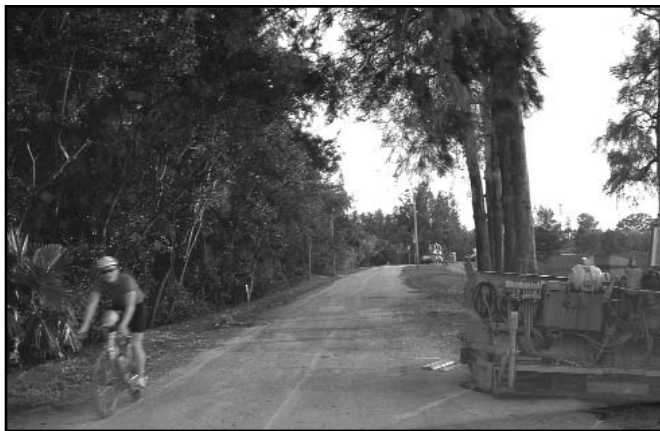
Rio Vista Trail under construction and being used before its open.
